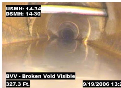
2-inch PE gas pipe cross-bored through an 8-inch sewer lateral.
