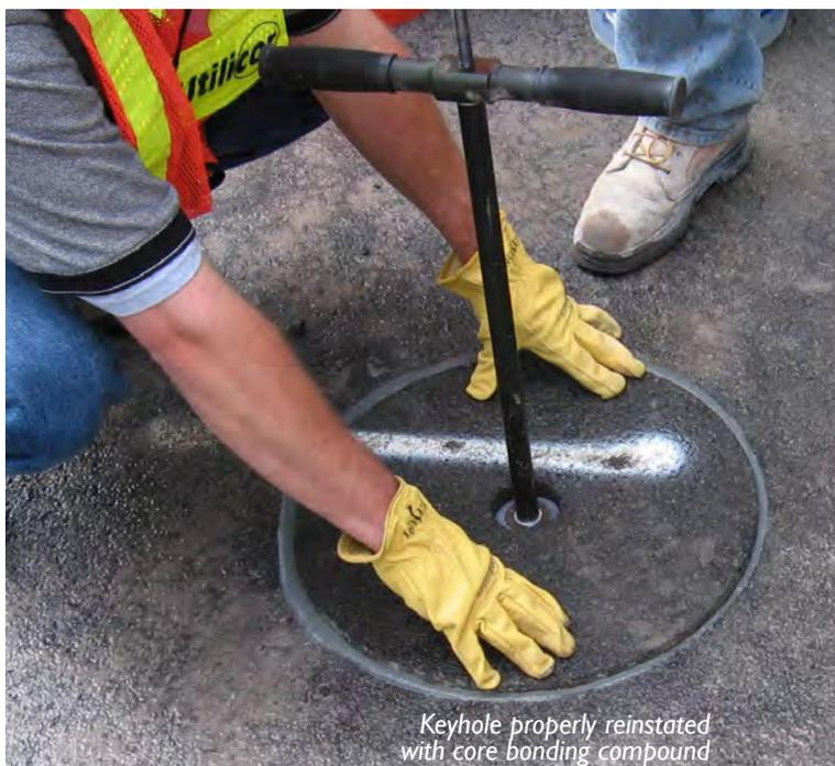
Keyhole properly reinstated with core bonding compound
