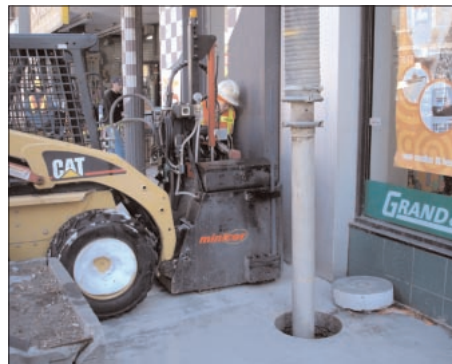
Keyholing technology helps to facilitate SUE work.
