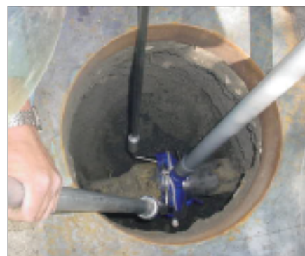
Here, a bell joint encapsulation is carried out with long-handled tools.
