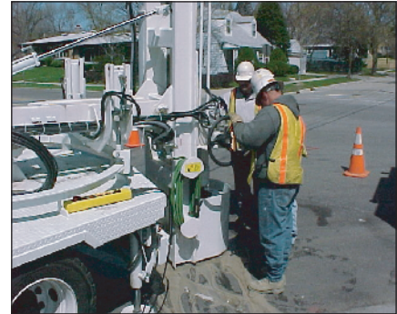
Bellwood's crew coring the roadway in preparation to repair a bell joint.
