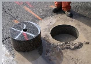
corners of the repair, as well as in the abutting pavement. It is these corner cracks, and the sawing overcuts present in most conventional cuts, that are the access point for ground water that is the major cause of premature pavement failure and potholes.
