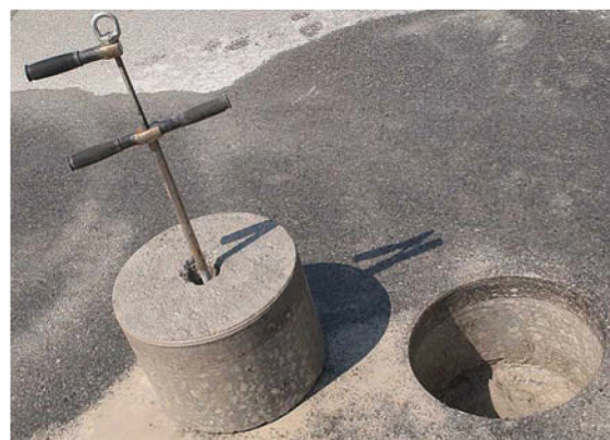
An 18-inch-diameter core is extracted from the roadway by a Utilicor keyhole coring drill at a hydroexcavation job site.
