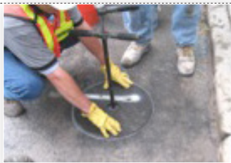
18-inch diameter keyhole core reinstated into pavement as a permanent repair.
