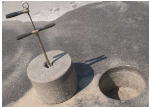
Left: Rotary coring unit cores 18-inch (457 mm) diameter core.
