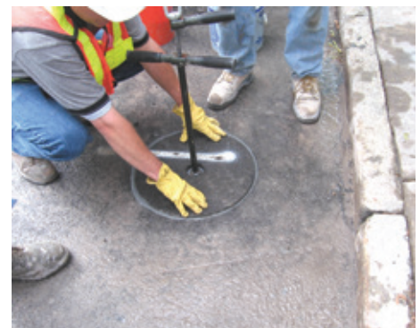
Centre: Core is removed and set aside. Vacuum excavation (not shown) is used to expose the infrastructure.
