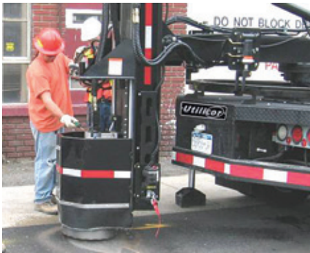
Left: Rotary coring unit cores 18-inch (457 mm) diameter core.
