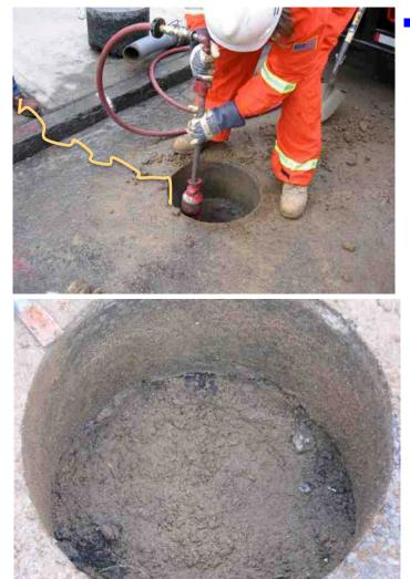
The hole is then back filled and compacted to the level of the base of the pavement so that the core or coupon of pavement can be reinstated.
