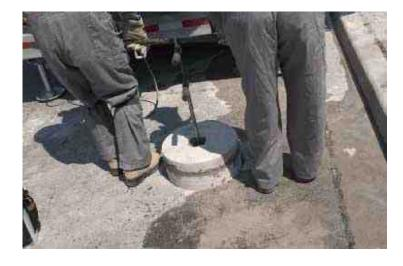
... the core is reinserted into the hole and fitted to the level of the surface.
