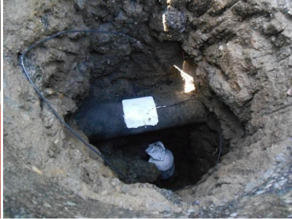
This shows the complete anode installation before backfilling.
