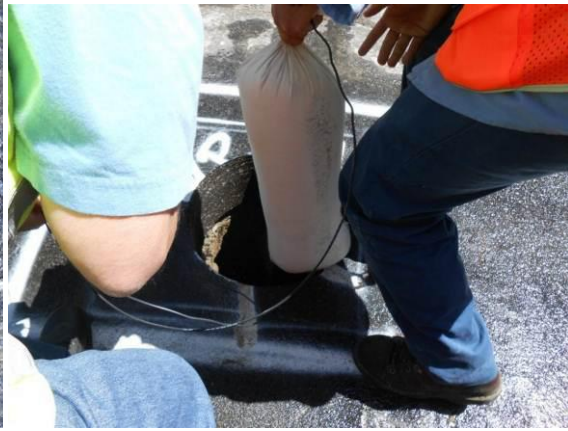
An LADWP-supplied anode was then placed in the hole.
