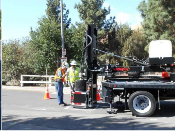
The coring rig positioned over excavation location.
