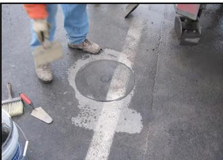
The reinstated core will begin to set up within 15-20 minutes. Take intermittent temperature readings to better gauge set time.
