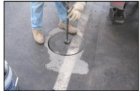
Remove the core heater and place the core in the opening, which will keep the core warm while mixing the Utilibond. Once ready, remove core, pour in mixed Utilibond, and reinstatement the core as per normal procedure.
