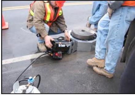
Place the core heater base in the hole and connect heater-blower to unit and place core on the base.
