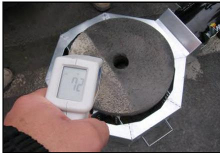
When the surfaces of the core reaches at least 70° F, the core reinstatement process can begin. Note: Make sure the Utilibond powder is stored in a warm location, and use warm water to mix with.
