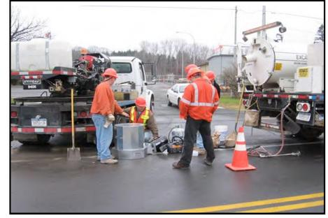
Place core cover on top of the Base, and open vents on top of core cover - ignite blower and position into baffle.
